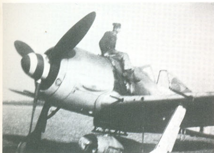
Some of II./JG 300's Fw 190A-8s like this one were fitted with four MG 151/20 cannon.
